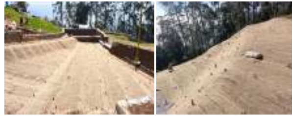
JGT is being laid out after backfilling the remediated soil
