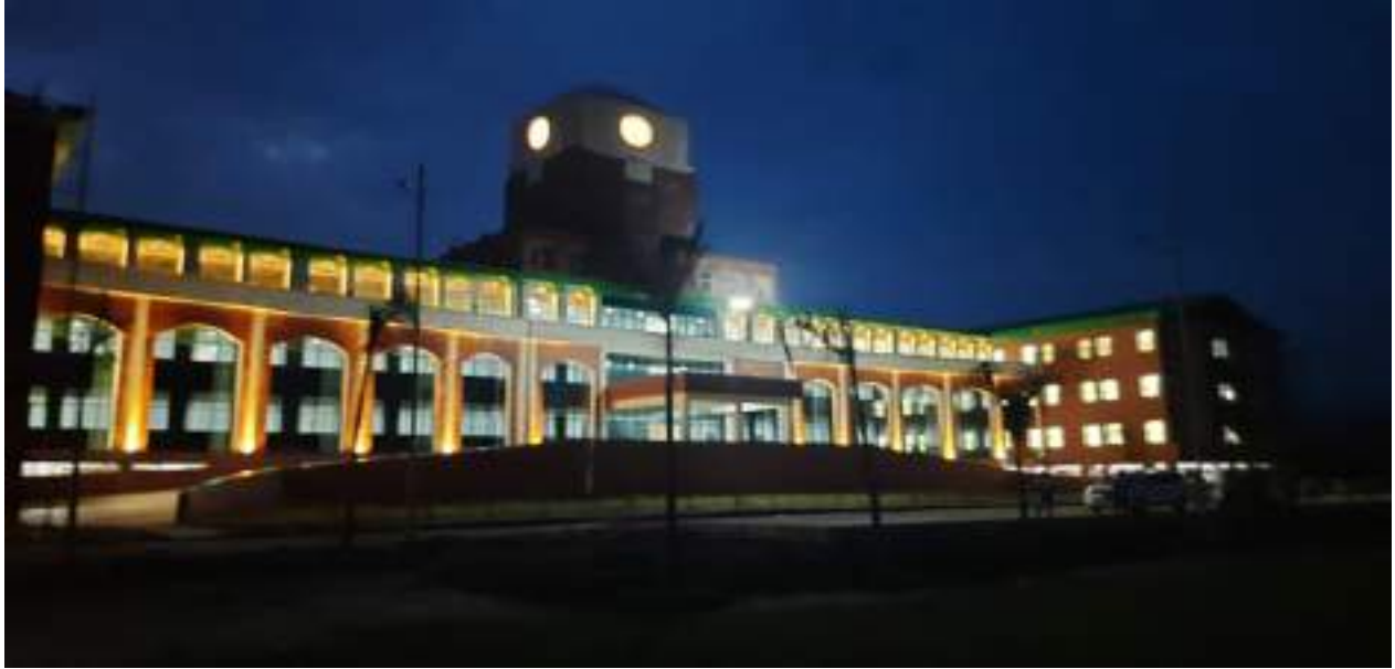
Night View of Admin cum Academic Building
