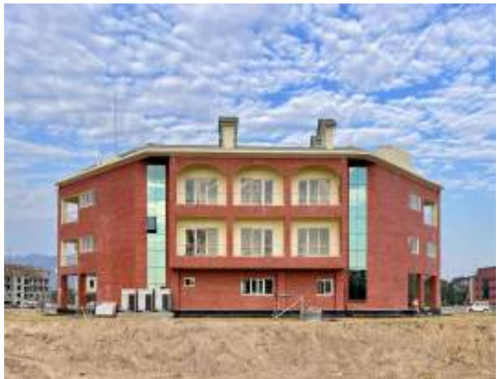
Guest house back side view
